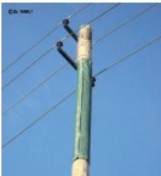
as a protection against woodbeckers on a telephone pole
