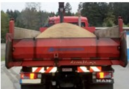
asphalt transport with jute cover
