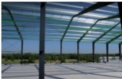
people safety net installed
